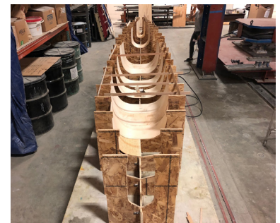
Figure 10: Interlocking skeleton with spacers being used during panel installation
