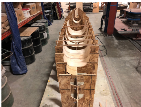
Figure 6: Interlocking skeleton with spacers being used during panel installation
