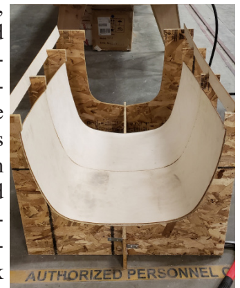
Figure 5: Mockup completed using plywood panels
