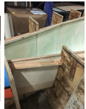
Figure 8: Installed braces to prevent bulging in panels
