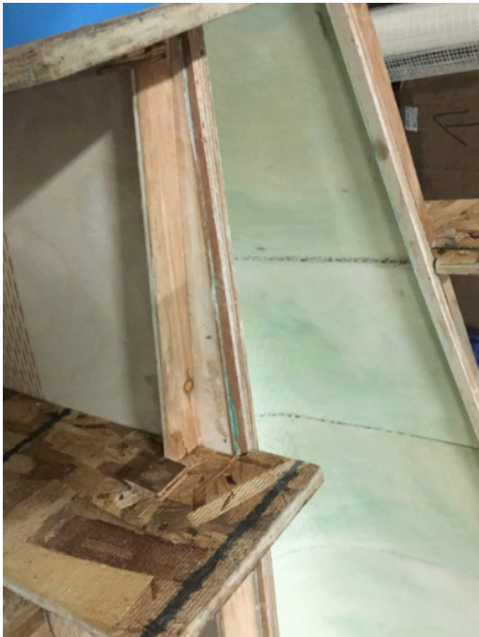
Figure 7. Installed braces to prevent bulging in panels
