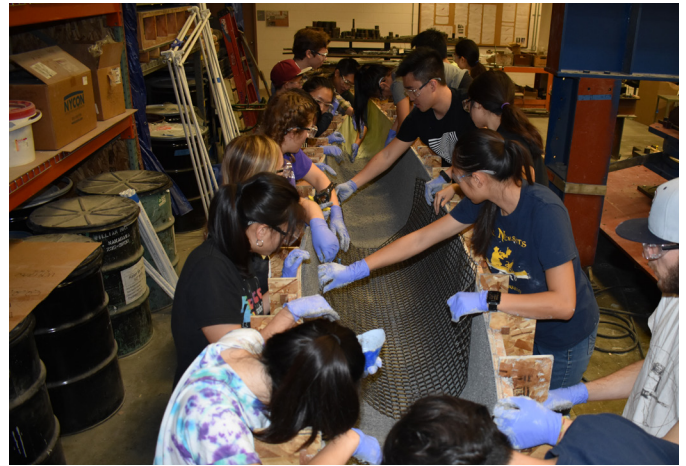
Figure 3. Basalt mesh installed during casting day
