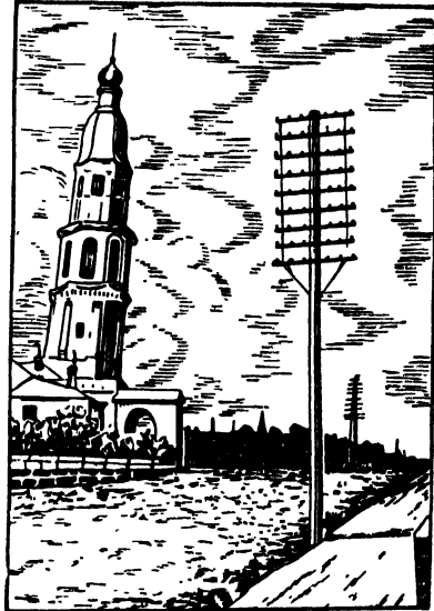
Fig. 15. Arkhangelsk leaning campanile. A reproduction from an old photograph
